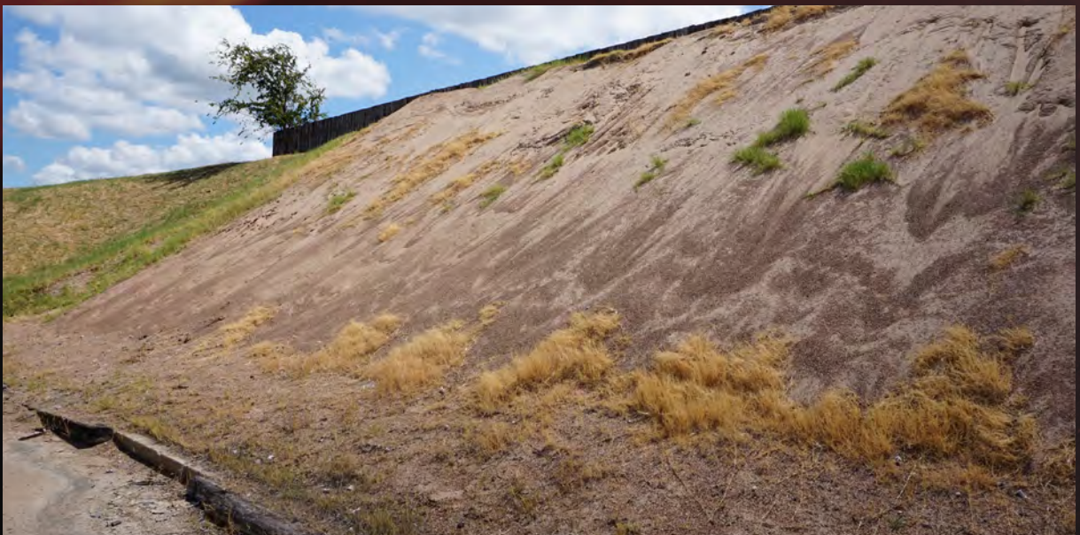
Existing dirt berm can be used as support for the STAPP EBC
